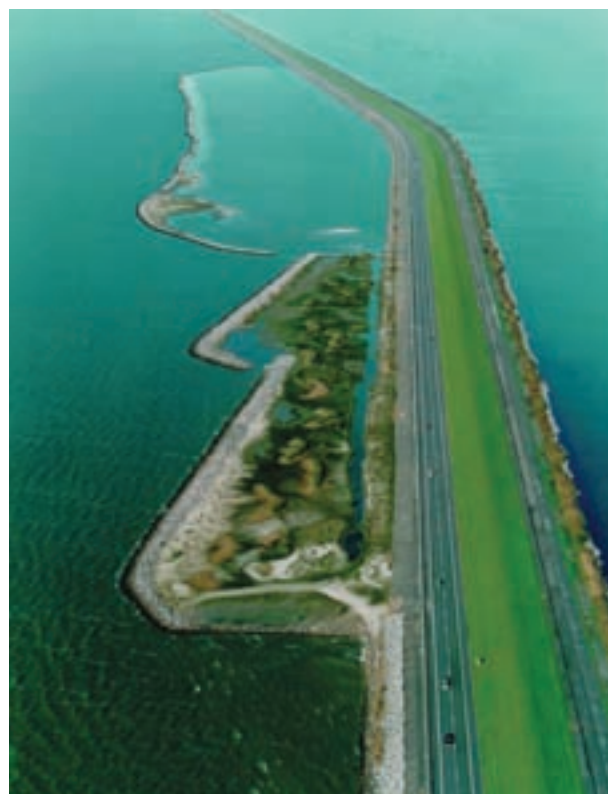
FIGURA 8. Dique secundario cuyo núcleo está construido con geotubos. / FIGURE 8. Secondary dam constructed with geosynthetic tubes as a core.
