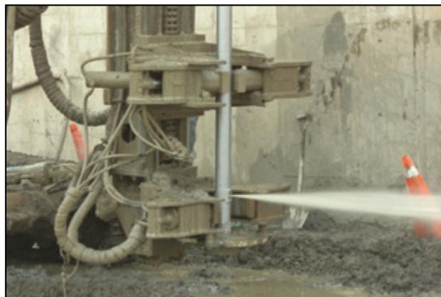
Figura 1. Detalle del chorro Jet Grouting (Pilotes Terratest S.A., 2011).
